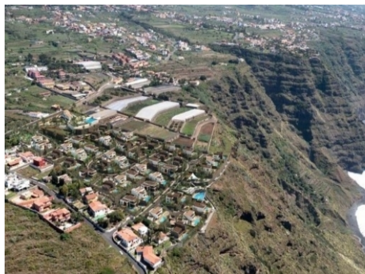
Nice views of the project
