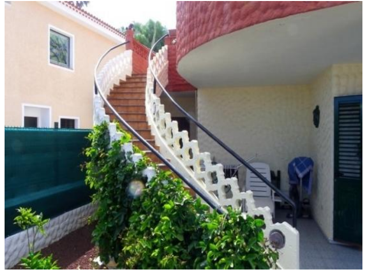
Curved exterior staircase
