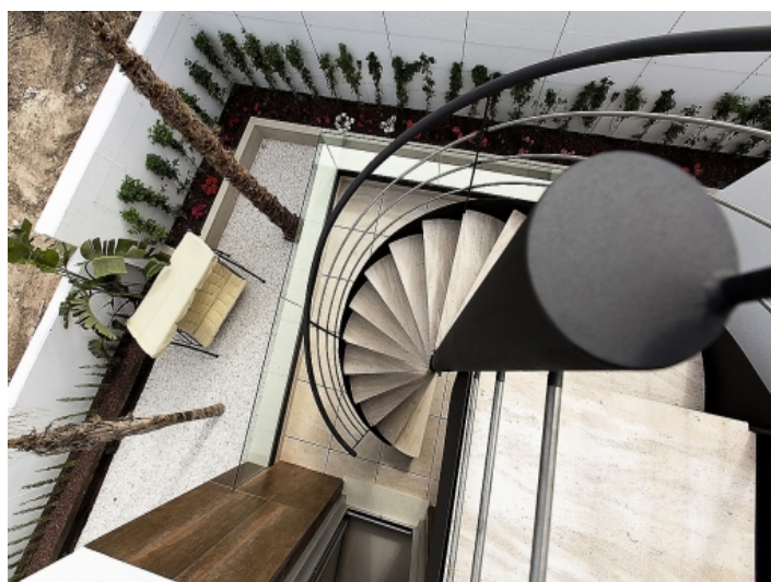
Spiral staircase to the roof terrace
