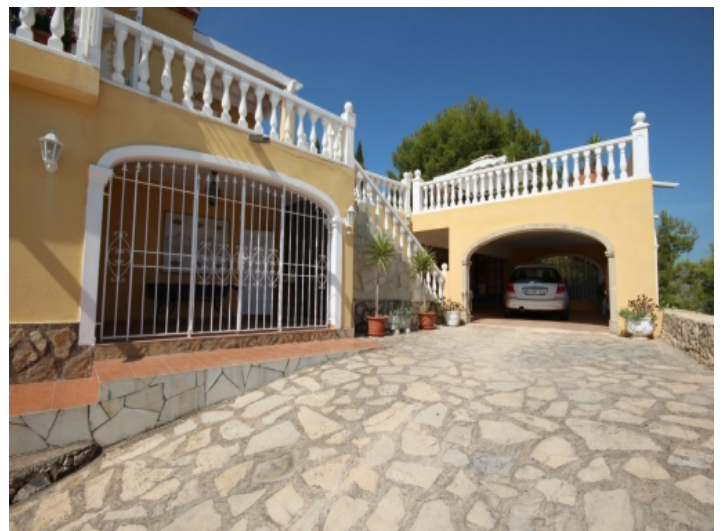
Entrance and garage
