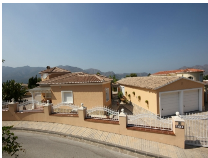
Entrance and garage
