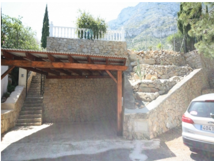
Entrance area and covered parking spot
