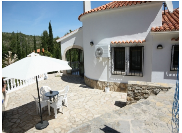
Terrace and side entrance
