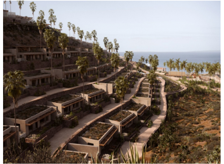
View to the complex
