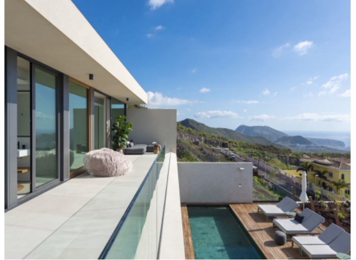
Balcony and terrace
