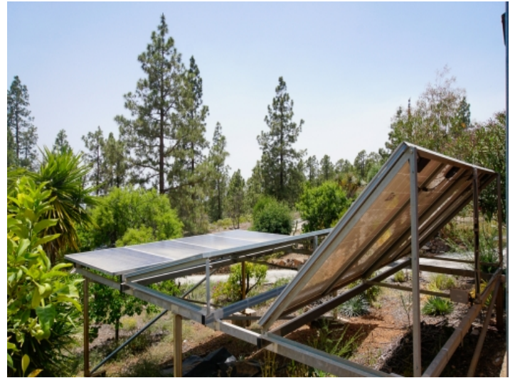
Large solar panels
