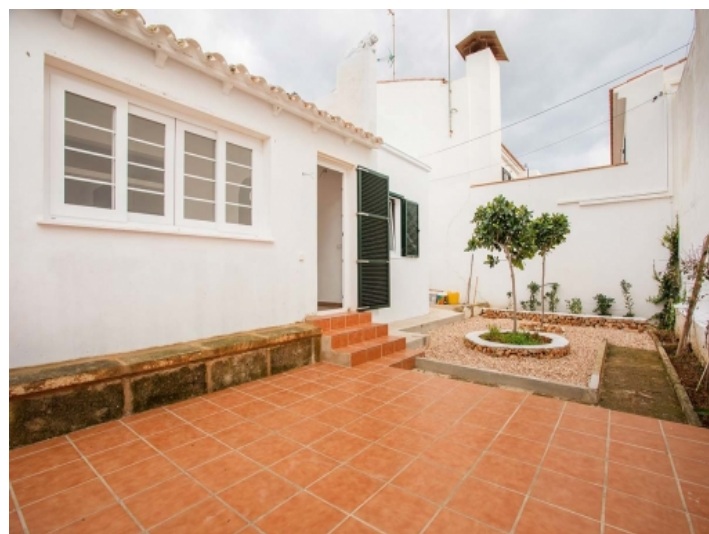
Front terrace and access to the house
