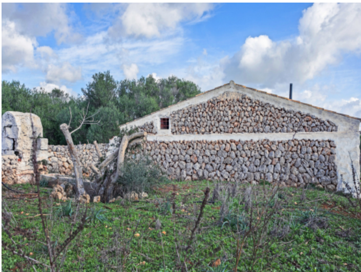
View of the stone facade
