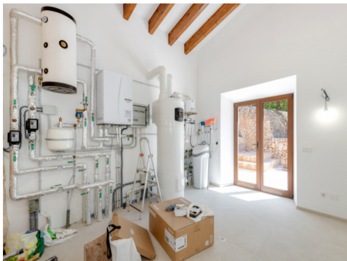
Storage and utility room
