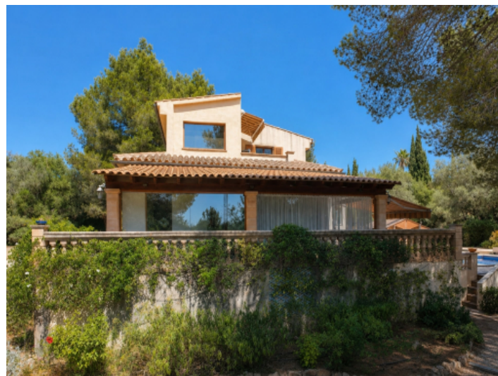
View of the finca from the driveway
