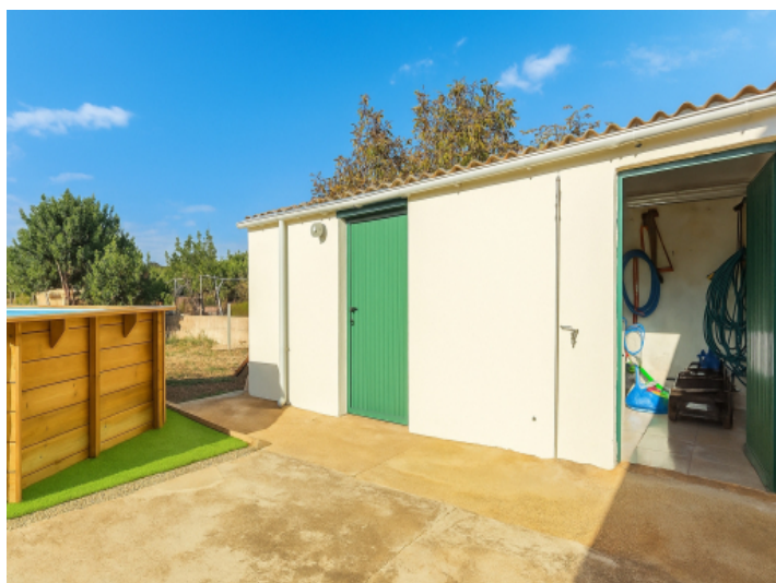
The swimming pool and the annex building
