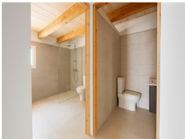
Guest toilet and separate shower room
