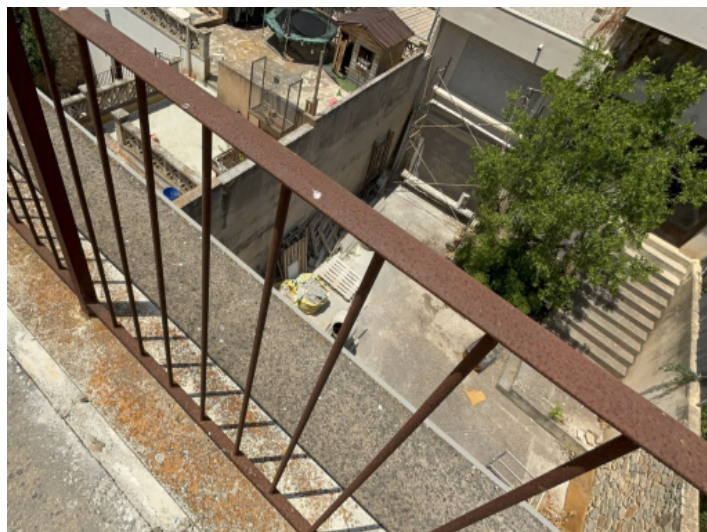
View to the patio
