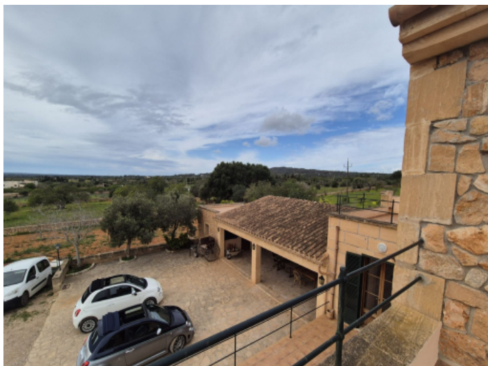
View to garage
