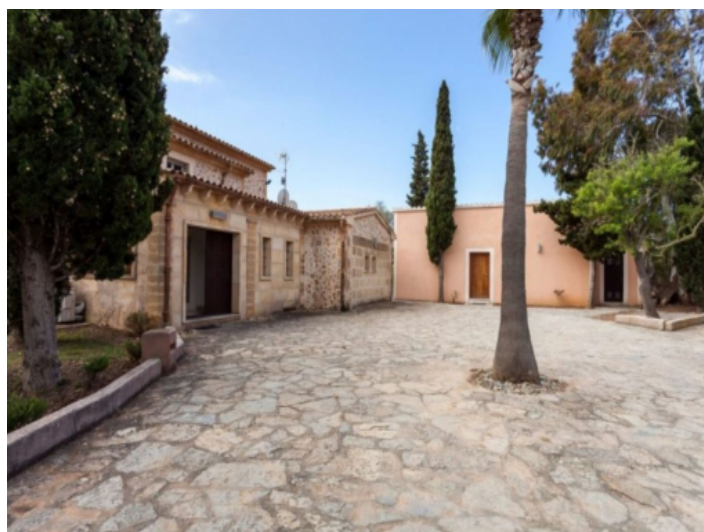
Patio and front façade
