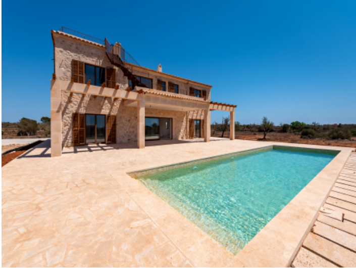
Facade and pool
