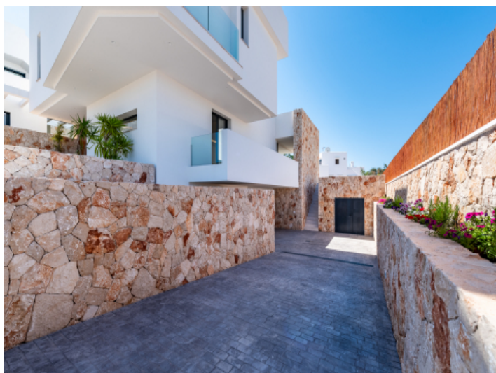
Access to the underground parking
