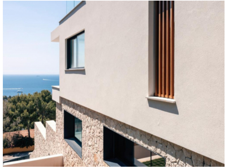
Lateral facade and views
