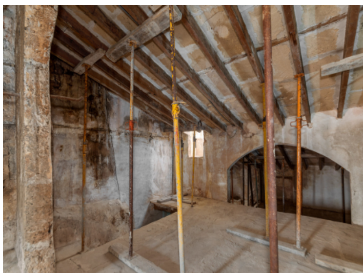
Original wooden beams
