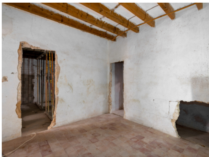
Old wooden beams
