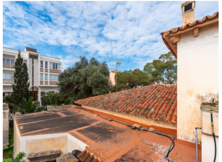
Views from the upper floor
