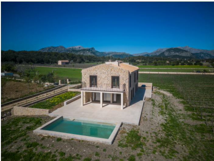
Aerial view to the property
