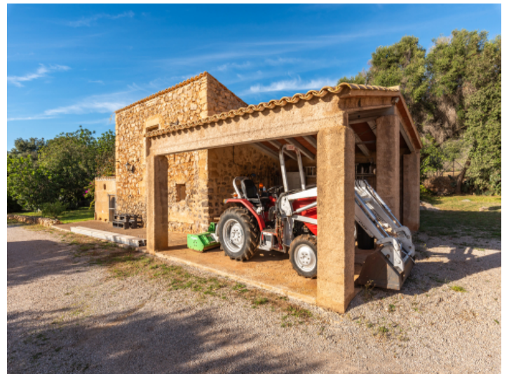
Carport built with natural stones
