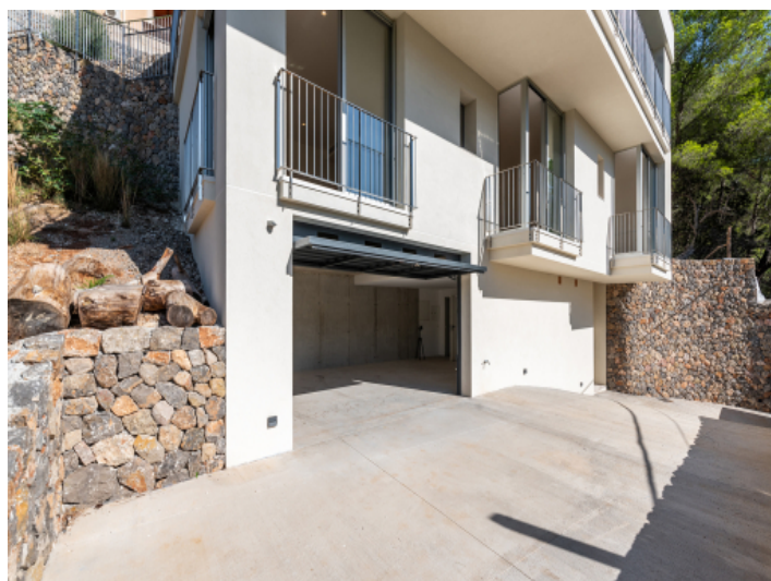
Access to the garage
