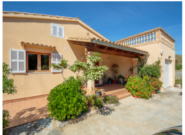
Access and front terrace
