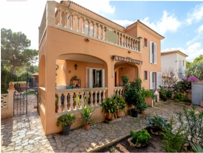
Exterior view of the house with 2 living units
