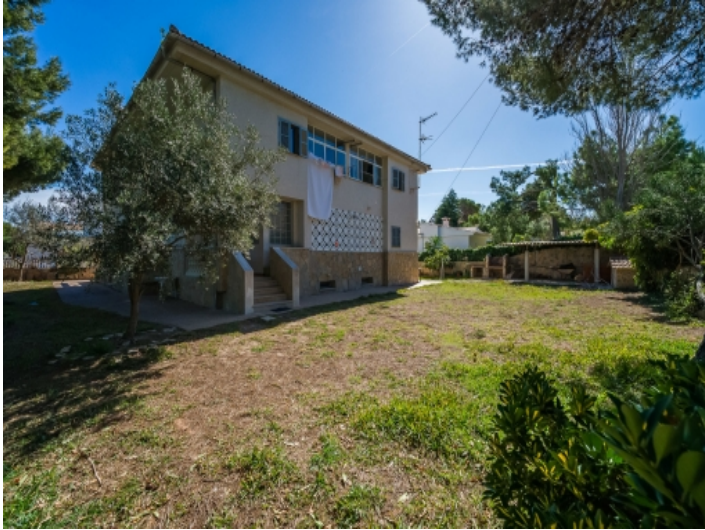
Exterior view of the house
