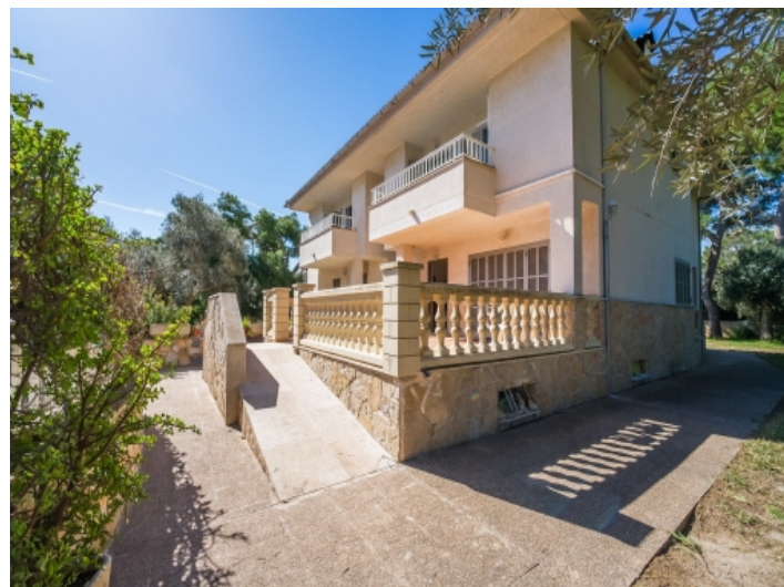
Sunny terraces and balconies
