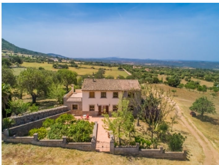
Exterior view of the finca
