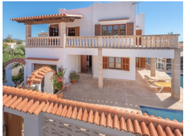
Front view and entrance to the house
