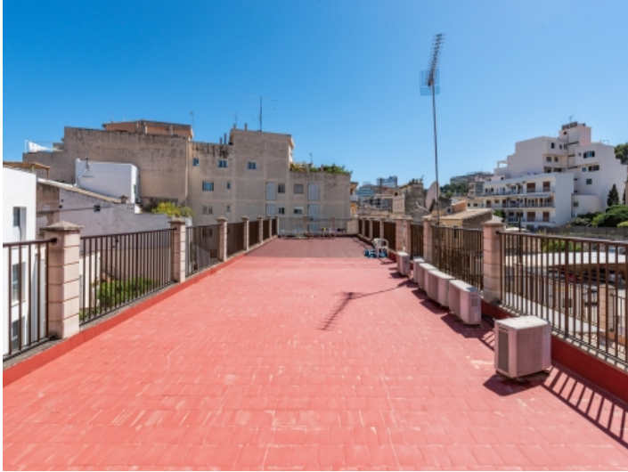
Extensive roof terrace
