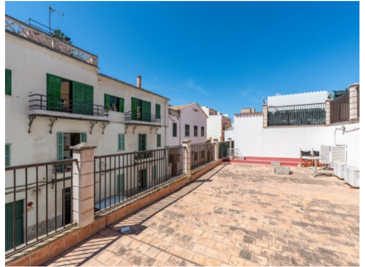
Lower part of the roof terrace
