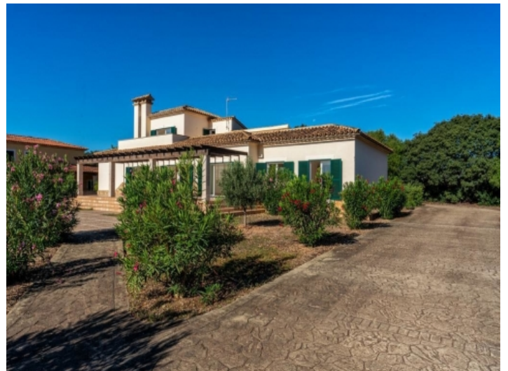
Access to the house
