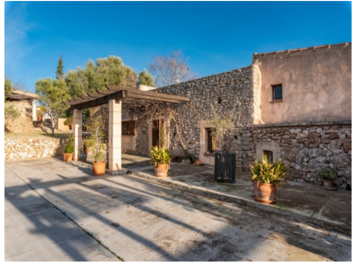
Front view and access to the house
