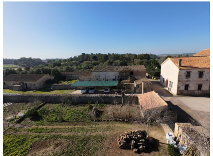
Covered parking lots
