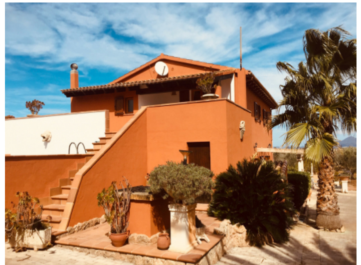
View from the south
