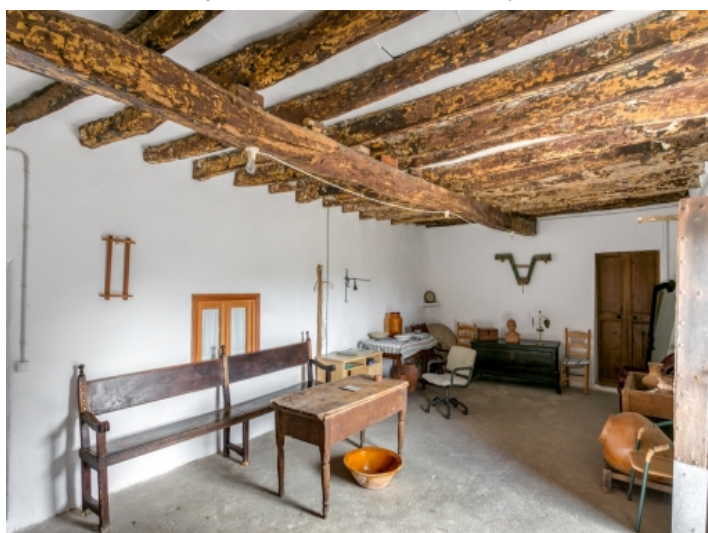
Room with wooden ceiling beams
