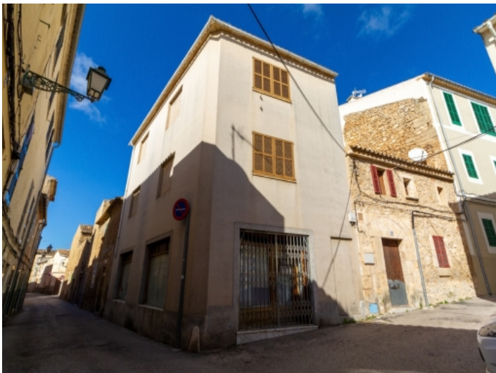
Exterior view of the second building
