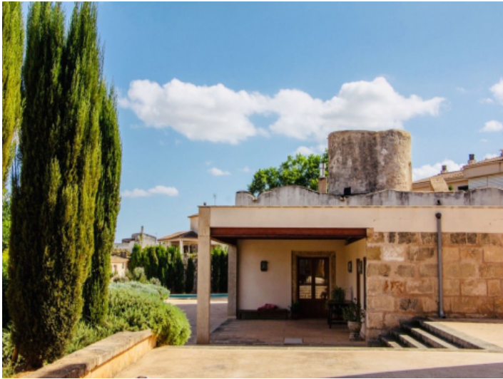
Completely renovated mill in the village of Llucmajor for June,
