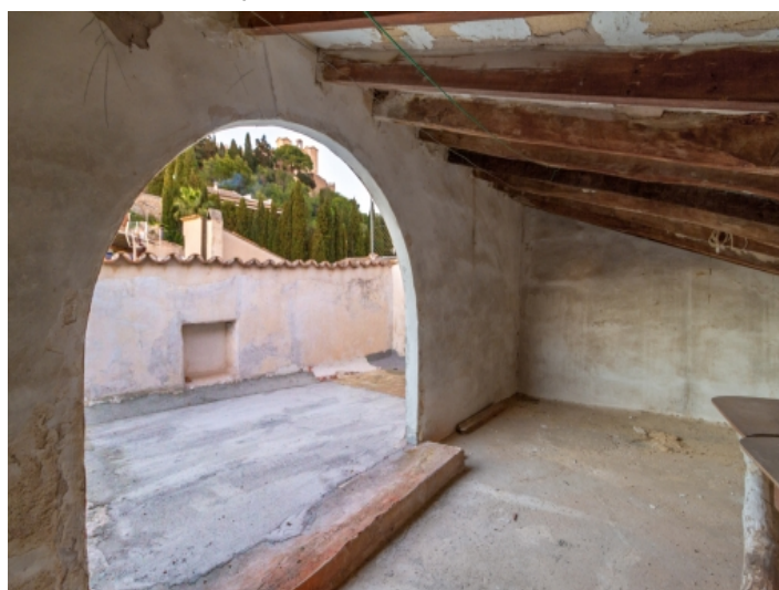
Additional room on the roof terrace
