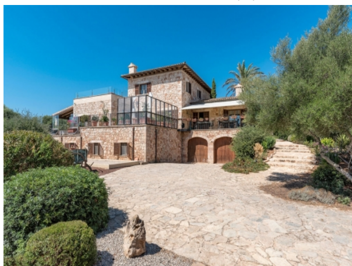
Front view of the finca with several terraces
