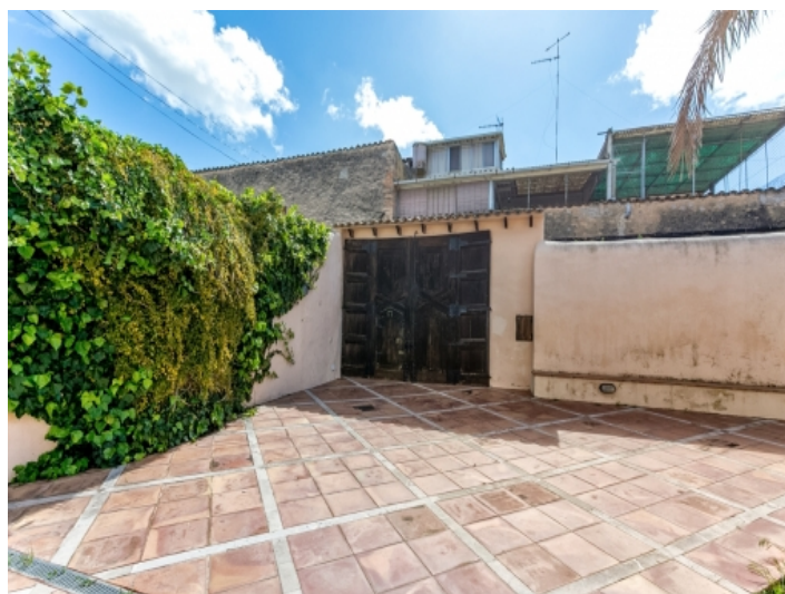
Entrance door to the plot
