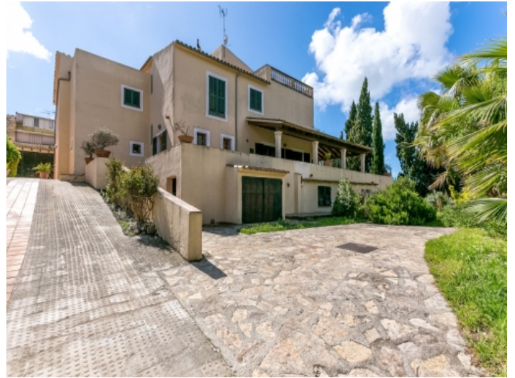
Rear view of the spectacular manor house
