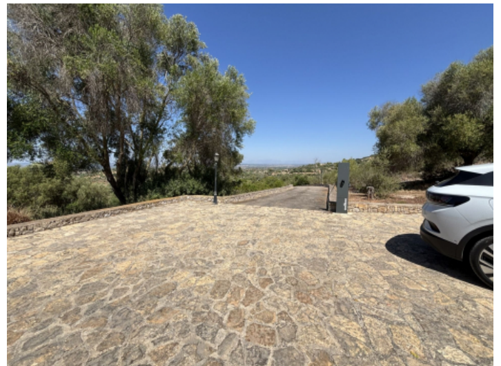
Parking spaces with charging station for electric cars
