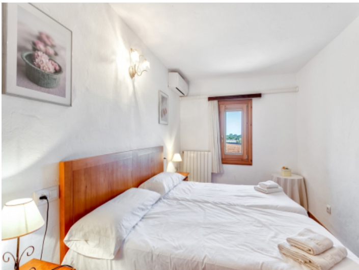
Air conditioning and heating in the bedroom
