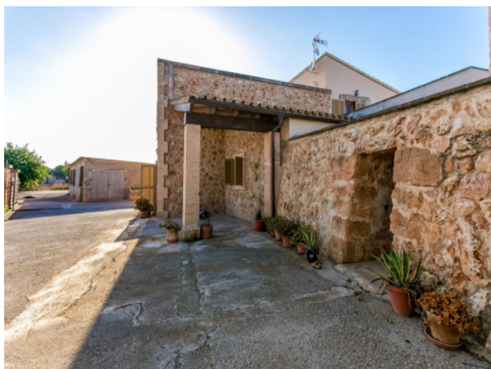
Typical natural stone walls
