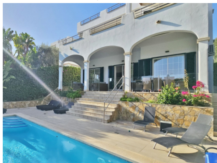
Covered terrace and sun terrace
