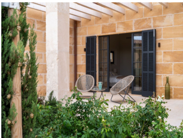
Façade partly covered with sandstone
