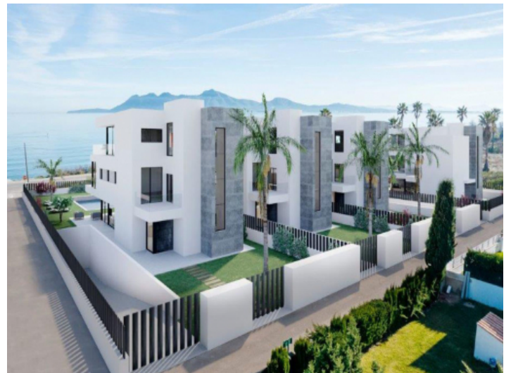
modern-architecture-front-sea-views-living-room-frontline-po rt-pollensa-new-buil-minimalist-villa-ensemble-four-villas-lle naire
