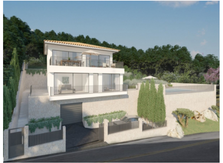
Exterior view from the street
