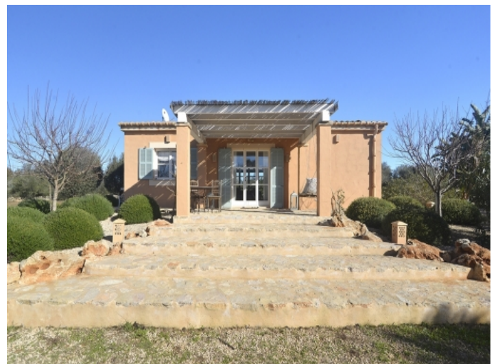
View of the guest house
