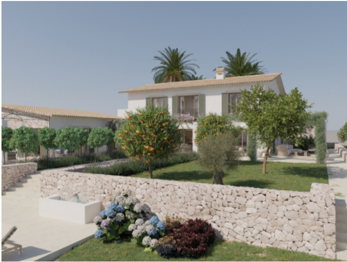
Front view of the newly built project
